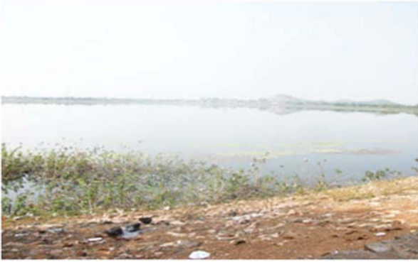
5. A view of Odar Dam, Vill- Tappa, Rajnandgaon(C. G)
